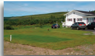
Completed peat system, Forteau, Labrador.
